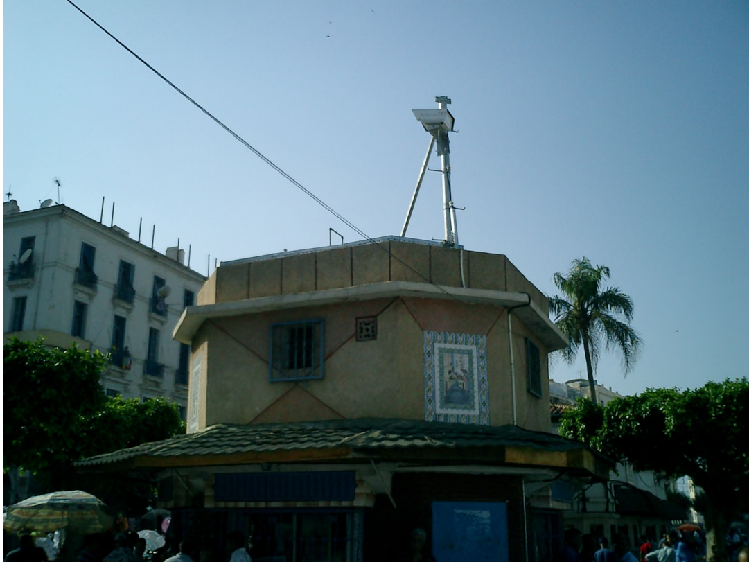
PAV's FSO link head in Algiers
