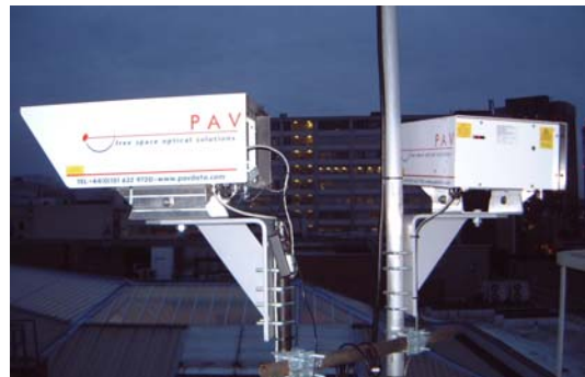
PAV's FSO links installed in Birmingham
