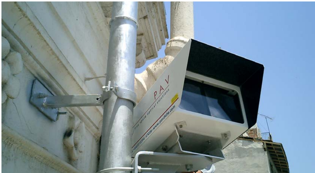
PAV's FSO link head during installation in Algiers
