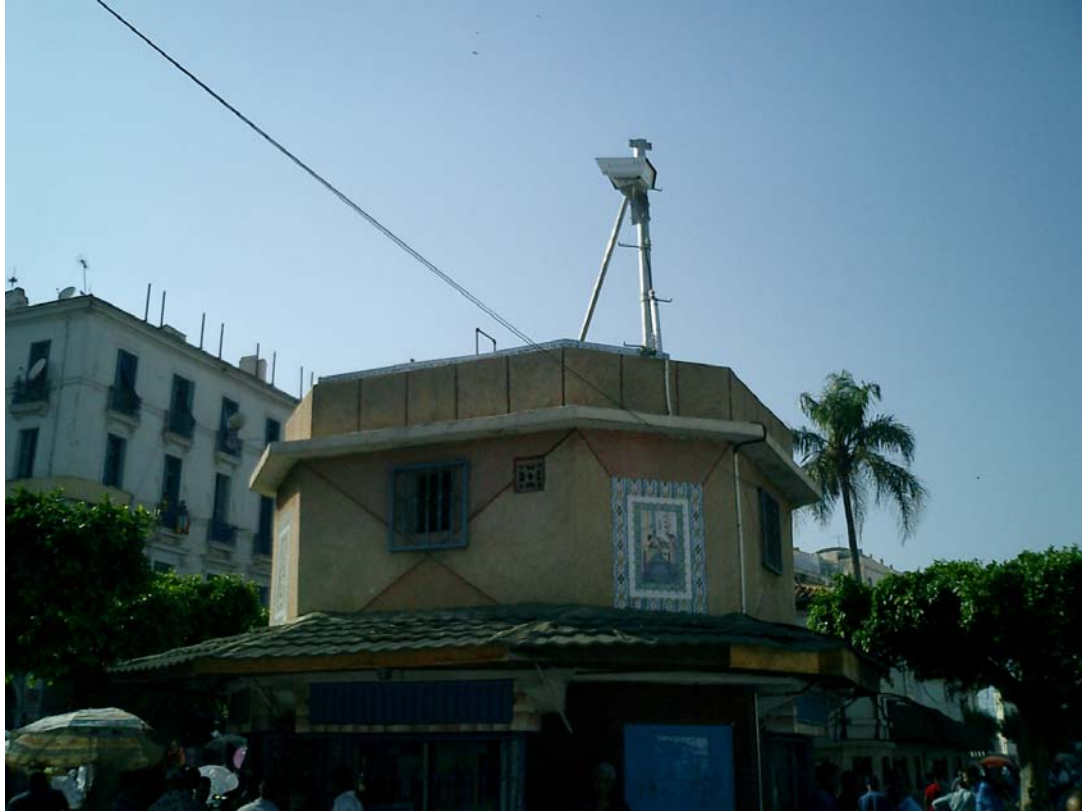
PAV's FSO link head in Algiers
